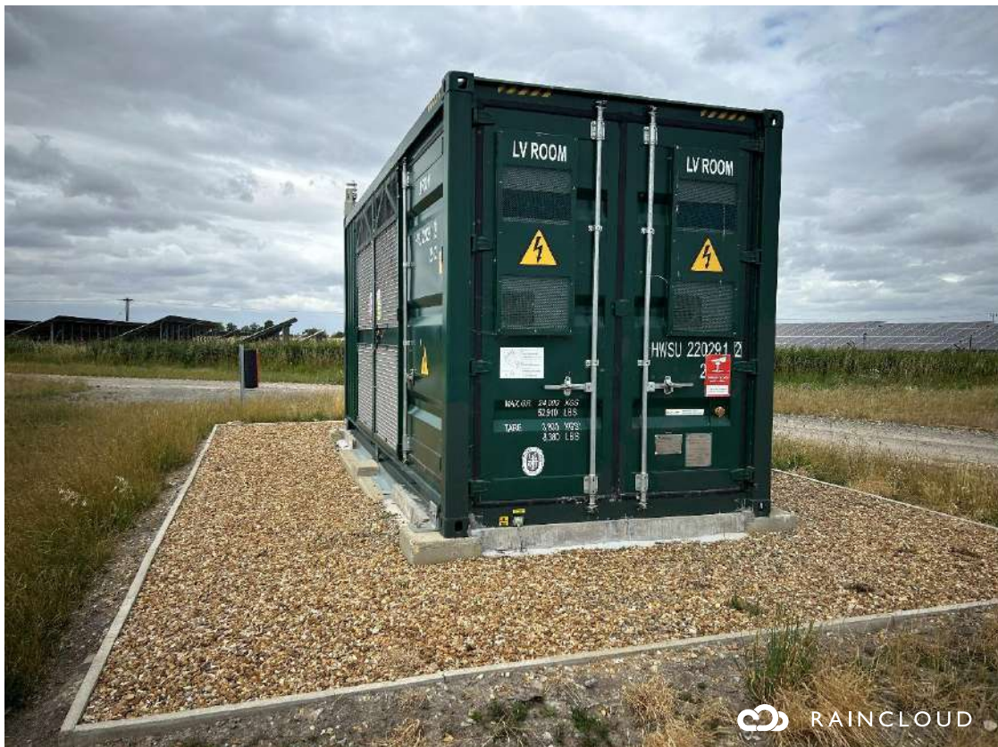
Plate 12-33 Conversion unit gravel surround
