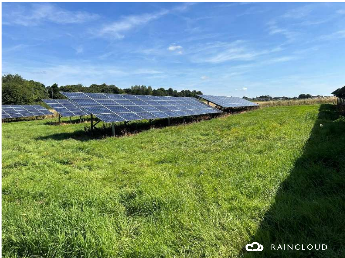
Plate 12-26 Established grassland and vegetation cover at a Solar Farm
